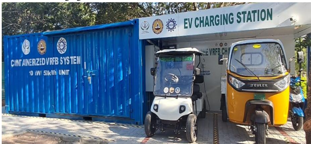
A photograph of 10kW/0.1MWh system developed with HEB for ONGC-Energy Trust Centre
